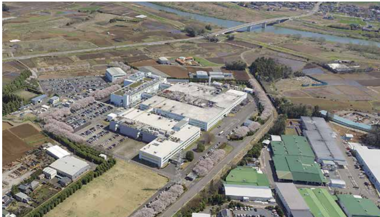
Tsukuba plant of Mitsubishi Materials Corporation in Japan, a strategic partner of MHT
