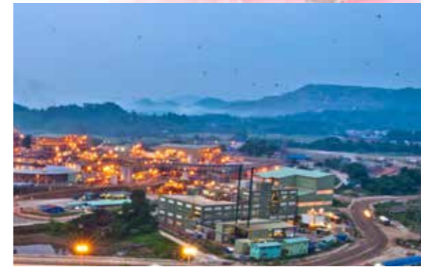
MTC's Hi-Tech processing plant
